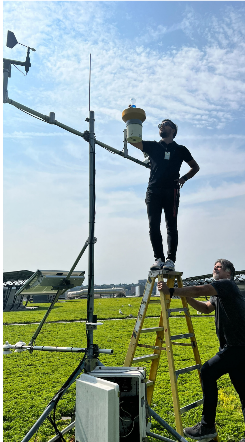
Green Roof Monitoring: CCRUN researchers (including co-PI Dr. Franco Montalto) conduct a tipping bucket test for rain gauge installed on one of the green roofs at the Javits Convention Center in New York City.
